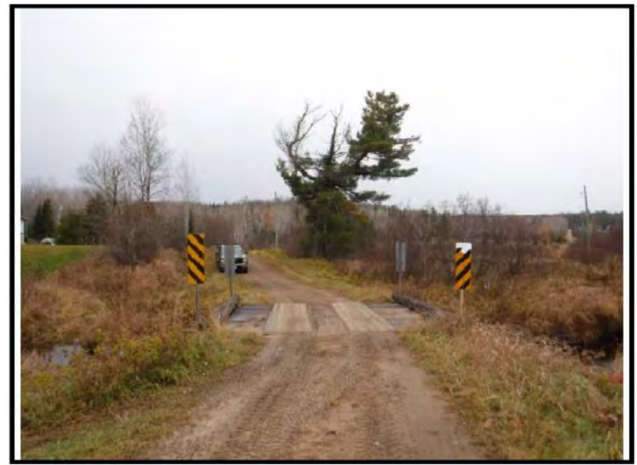
Photo 2 Structure from west approach
