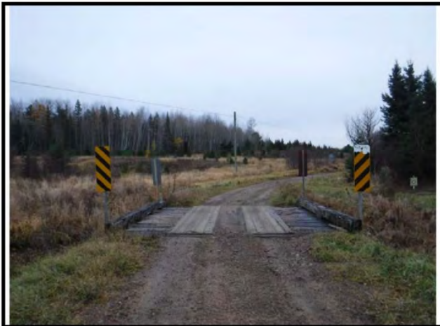
Photo 1 Structure from east approach
